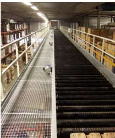
The bridge goes straight through the old warehouse.
